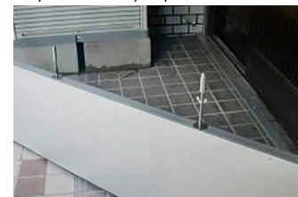
Example: Removable aluminum water stop in the entryway of a home
